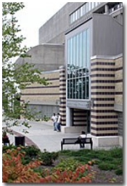
The Transition Academy at CCRI is located on the Community College of RI Knight Campus in Warwick, RI.
